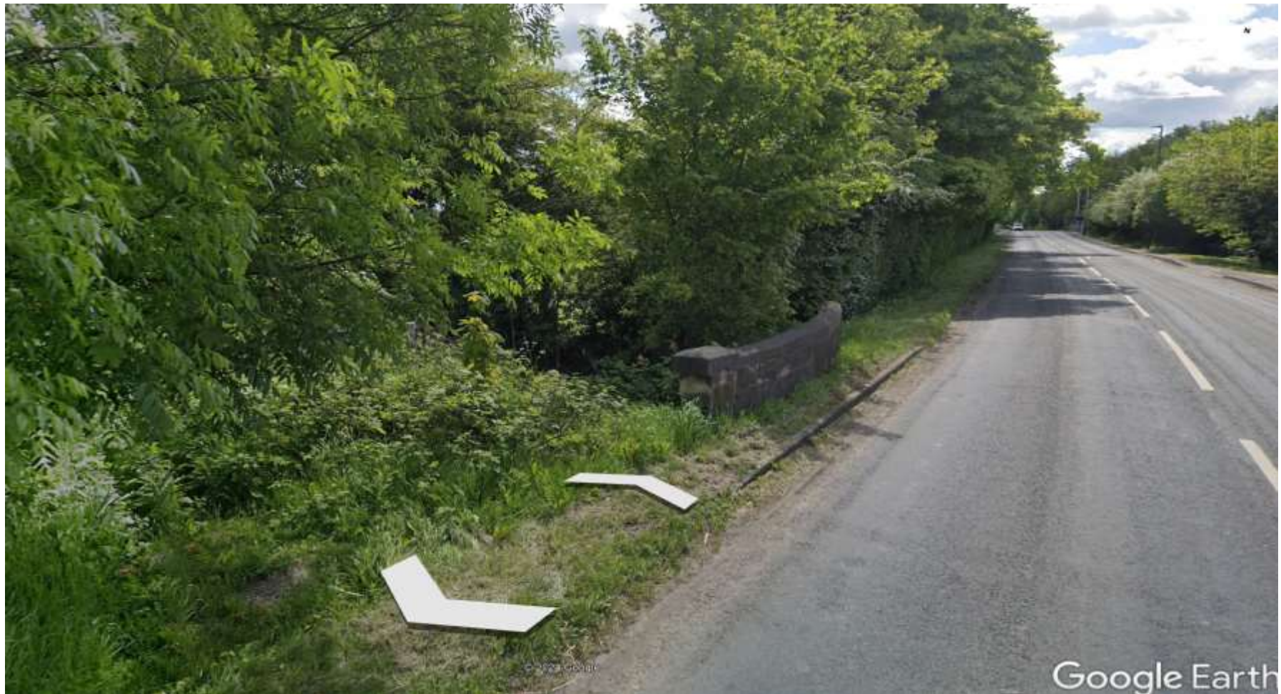
C - Image showing view of entrance to car park A from the North
