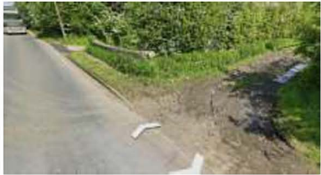
A – View of Exit of car park A from the South
